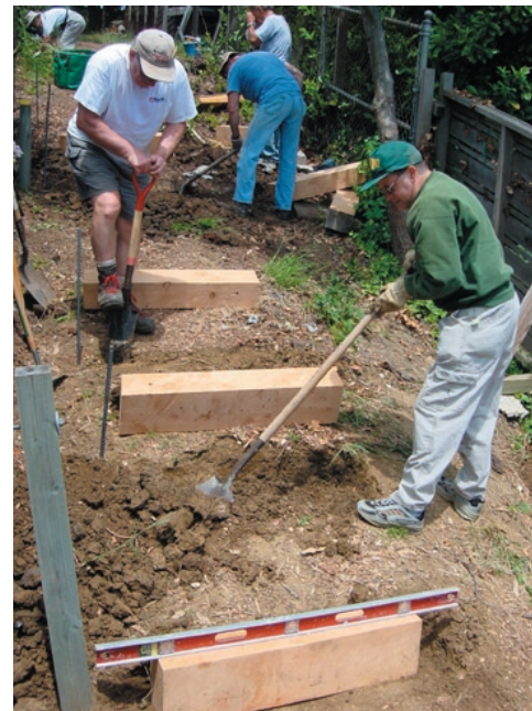
Neighbors and Berkeley Path Wanderers Association members added steps to the middle section of Stoddard Path on July 19th. This followed three earlier work parties over the last couple of months. Transformation has been amazing. When CalCorps students arrived for the first work party they looked uphill at a mess of ivy, weeds and tangled berry bushes.
